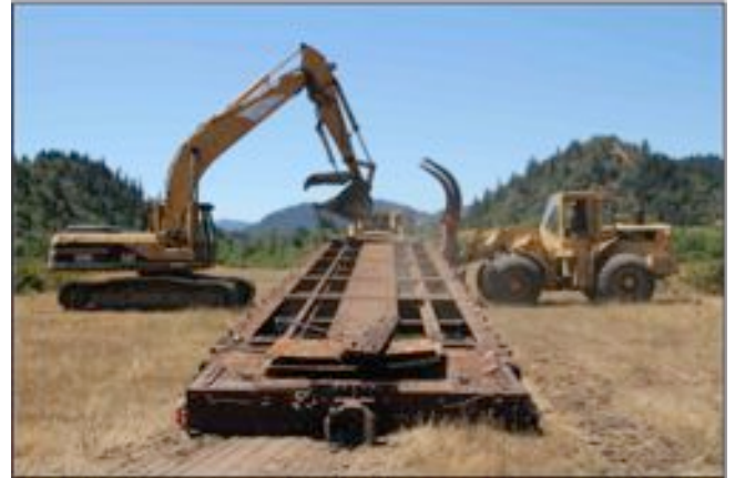
Above, the Museum brought a former Southern Pacific flatcar from Northern California. Below, volunteers created a virtual window to watch passing scenery.
