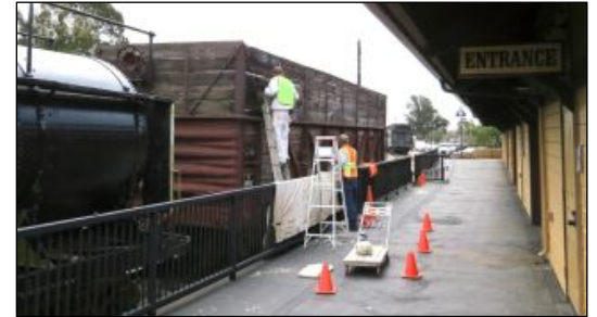
Painting contractor Greg Jackson (on ladder) and curator Brad LaRose start the effort with protective items, paint mixing, and brushwork.
