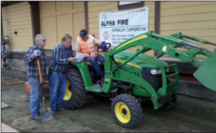
Tom Cooper, Ted VanKlaveren and Howard Amborn go over the plans for leveling the display track by the Freighthouse. Photo by Gary See
