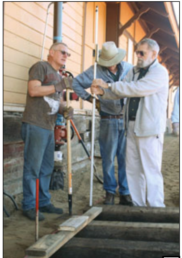
Tom Cooper, Chris Hurd and John Marchetti determine the alignment of the display track. Photo by Gary See
