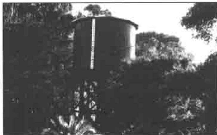
Newly restored water tank.
