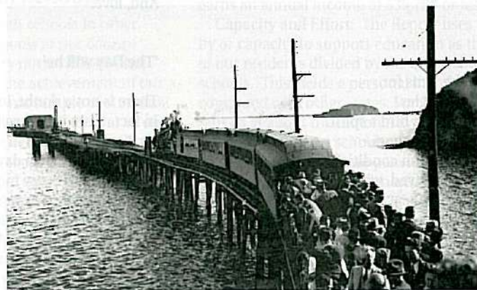
Central to economic viability of the Pacific Coast Railway was Harford's Wharf San Luis Obispo Bay where the line's passengers and freight connected with steam ships. This fact was not lost on these 1938 Railway Boosters as their 30-inch gauge train steams out on the wharf.
