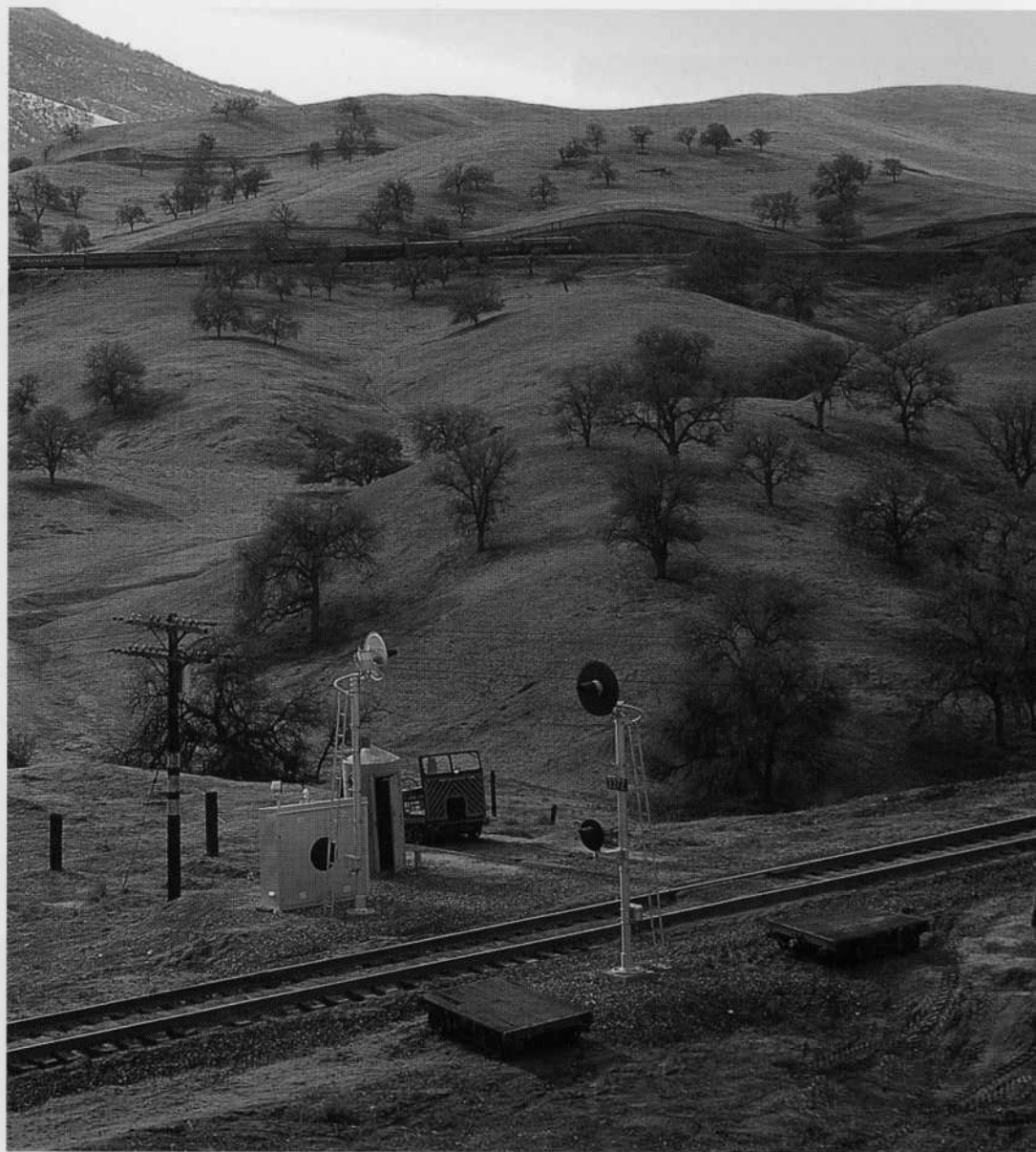
A familiar scene: A track inspector has set off his speeder at MP 337.2 in the Tehachapi Mountains between Caliente and the old siding of Allard, and awaits the passage of train No. 52, the San Joaquin Daylight about 1961. The ever-present concrete phone booth is close at hand. The door is open, and after No. 52 passes, the inspector will step inside to confer with the dispatcher about his next move. - R.O. Stolzenfels
